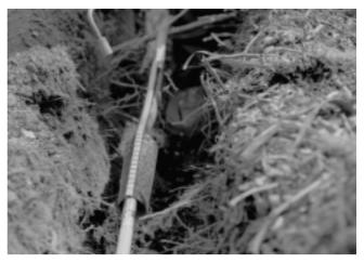
The CWST sleeve is simply wrapped around the damaged cable area and shrunk with a standard jointer's torch.
